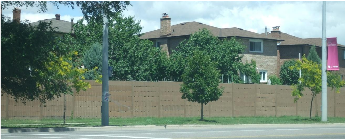
Highway 7 at Bruce Street
