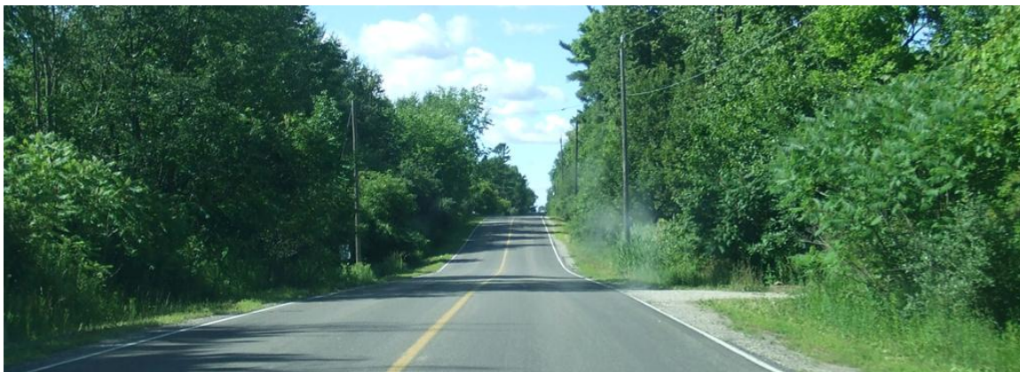
Pine Valley Drive at Major Mackenzie Drive
