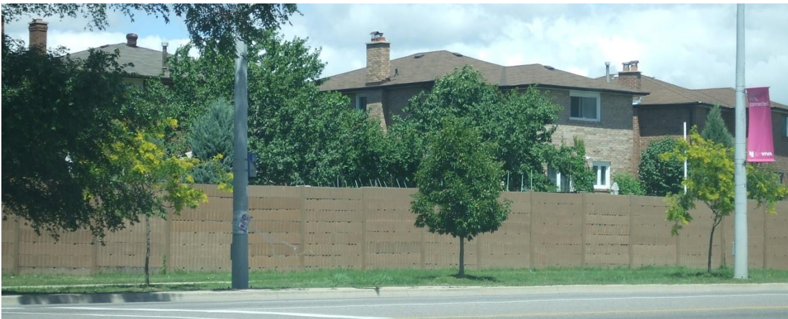
Highway 7 at Bruce Street
