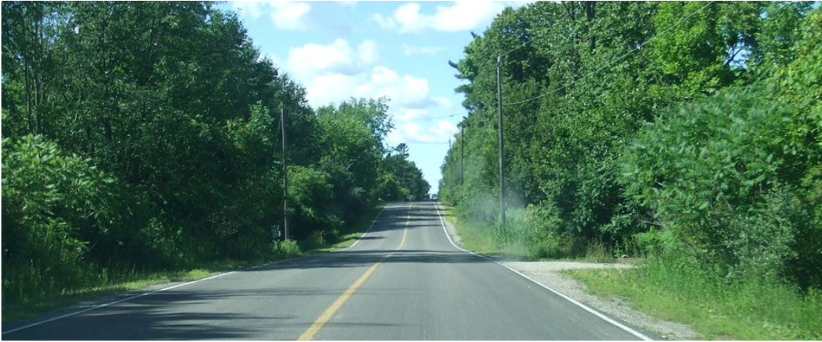
Pine Valley Drive at Major Mackenzie Drive
